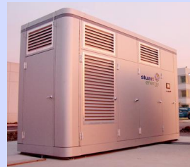
Hydrogen production Electrolysis Compression Storage and Dispensing
