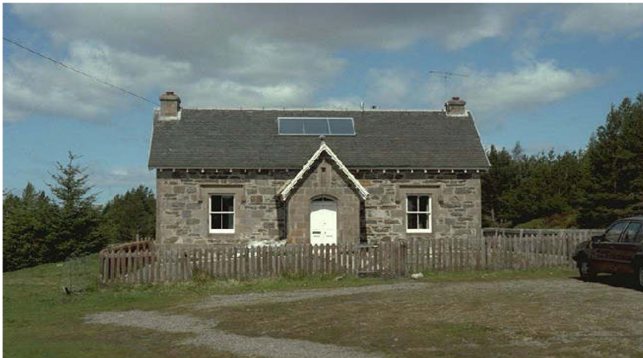
3 SQUARE METRE DOMESTIC SOLAR WATER HEATING SYSTEM
