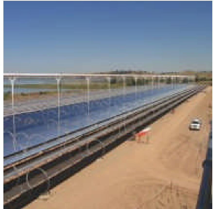
Liddell Power Station, NSW
