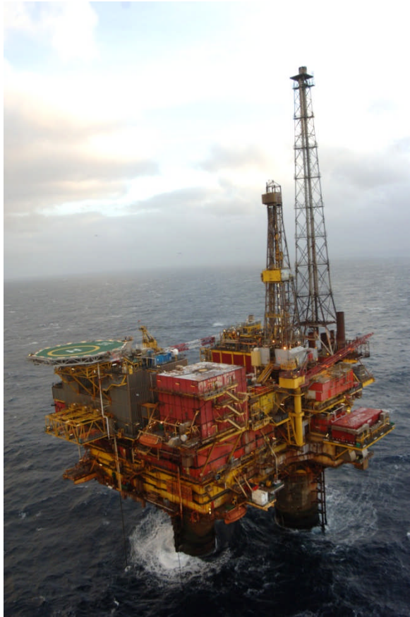
Existing oil platform, North Sea
